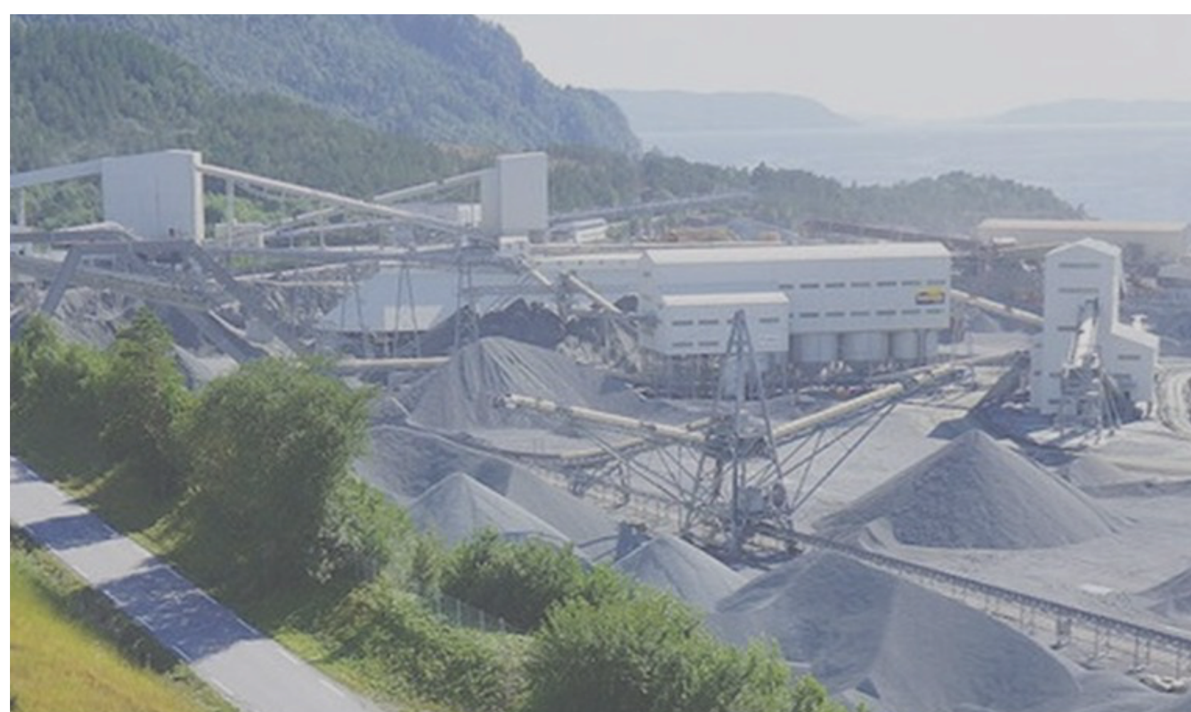
Photo: Jelsa Quarry in Norway using warehouses to enclose a portion of its processing facility.
